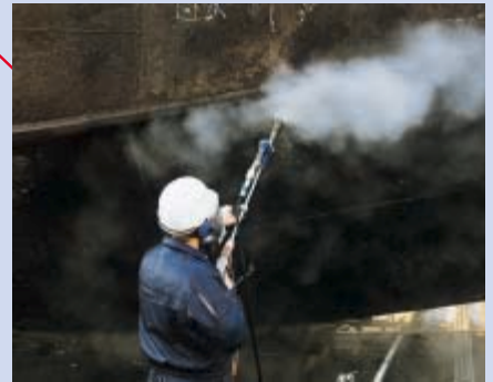
Weld seam cleaning and scale removal with the 3000-bar Modular Gun System .
