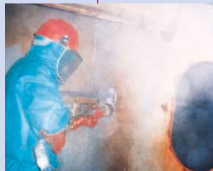
Ballast tank cleaning with the 3000-bar Modular Gun System .
