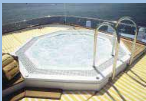
Addition of a new jacuzzi in sundeck redesign. In this case pipe work had to be incorporated in to the existing structure.
