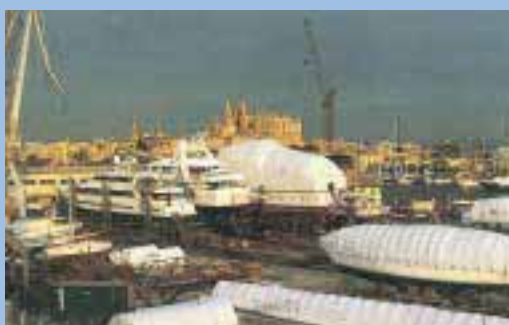
Topside repainting carried out under custom shrink foil covers protecting both the working area and the environment.
