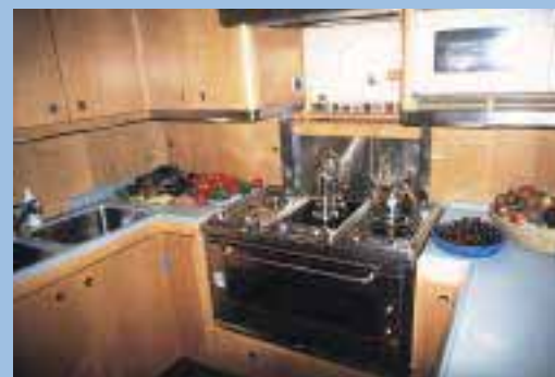
Galley redesign and modification to incorporate new appliances finished with Corian and stainless steel custom cabinets, all made on site.
